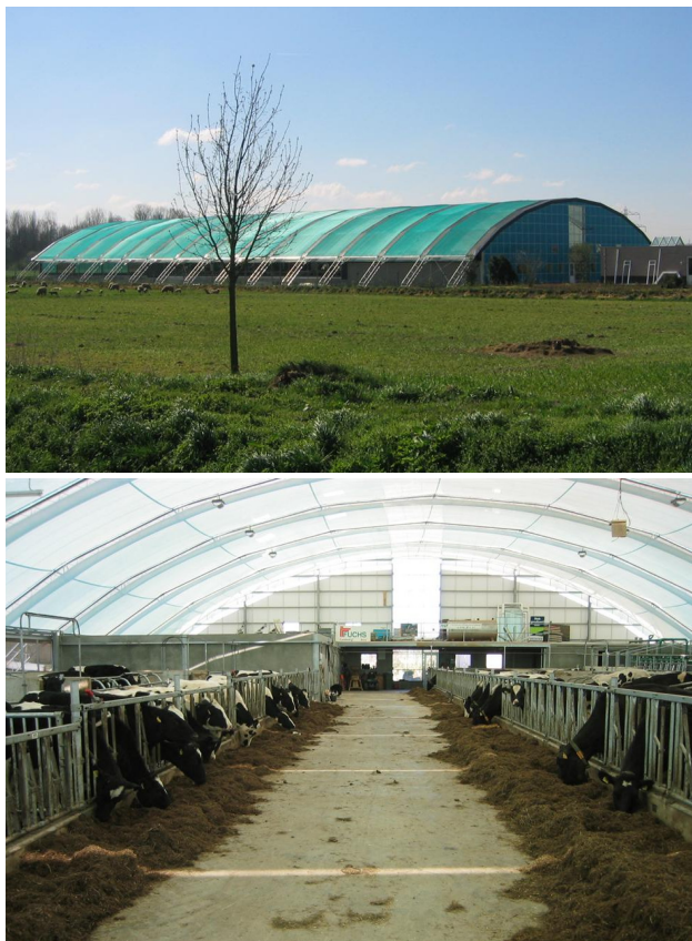
Figure 11 A & B Pilot project Arched Stable for dairy cattle in Dieteren, The Netherlands
